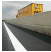
The advantages of the step profile compared to other shapes such as the New Jersey profile is to prevent the possibility of roll-over accidents and to significantly reduce vehicle damage and occupant injury.
