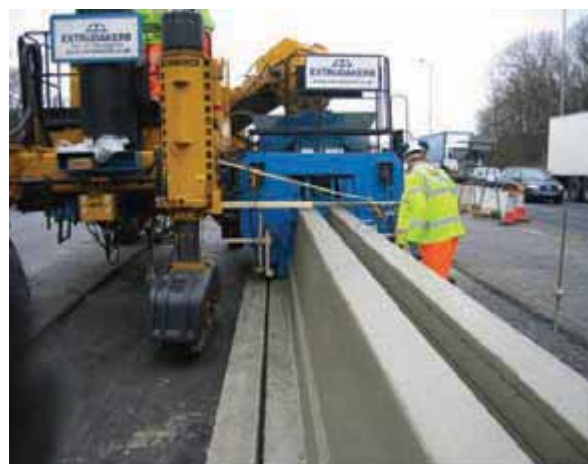
Figure 2.1: Wide profile CSB with integral cable trough.
