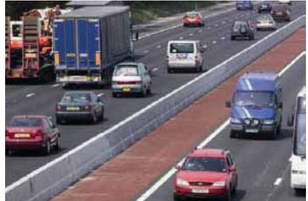
Figure 2.1.1 Concrete Step Barrier.
